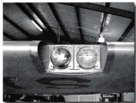
Existing Left Lights
